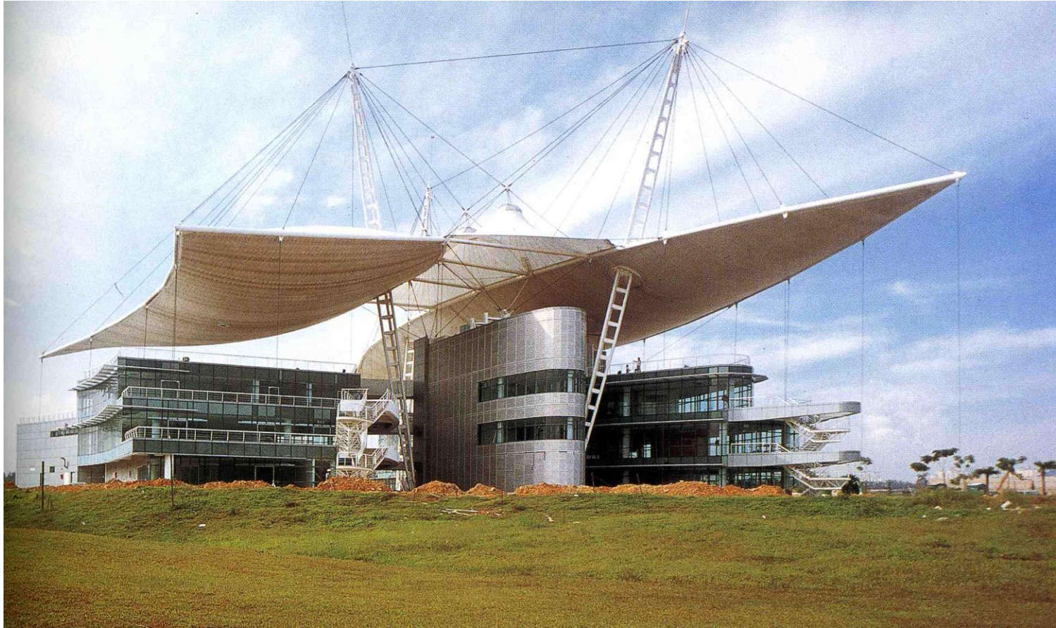
The Guthrie Pavilion; Shah-Alam, Malaysia, Ken Yeang, 1998
